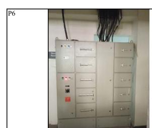
Shifting of 160A Electrical Distribution Panel (Quantity - 1 Nos.) with providing additional cables (Al and Cu) whichever required, Perforated tray (450\*50), Earth wires of 16 SWG with necessary miscellaneous items like lugs, ferrules (Al/Cu), glands, etc. with breaking, fixing and repainting of breaking area required for panel shifting.
