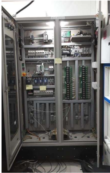
IloT Panel and WaterTreatment Plant Scale down model for ICS-SCADA Cyber Security
