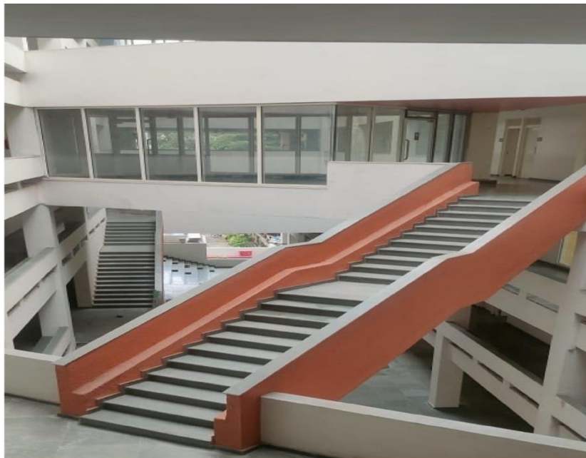
PG HOSTEL ATRIUM
