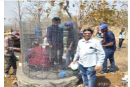
Ferrocement Tank Construction Workshop – Koshte Village
